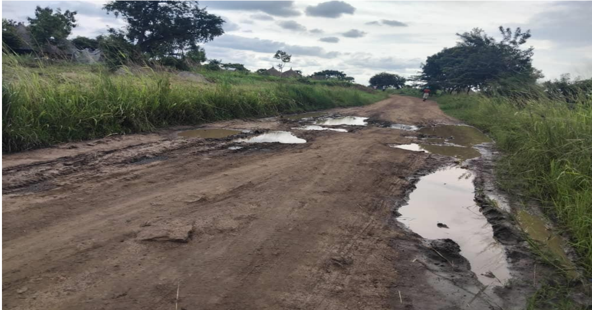
Figure 9: An almost road at Zone 1, block 2
