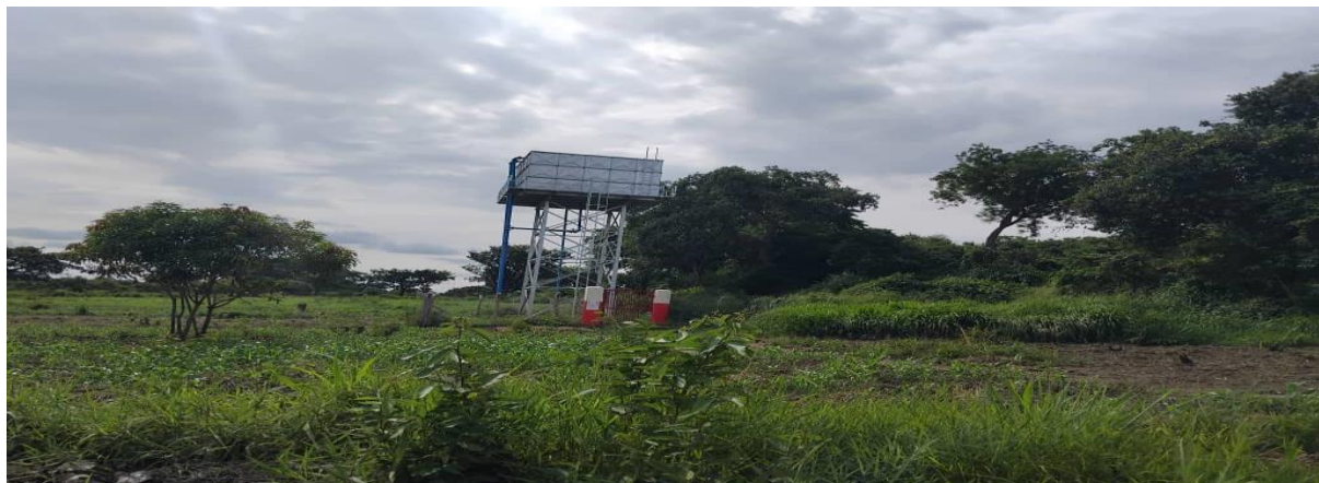
Figure 7: Water storage tank serving the settlement community.
