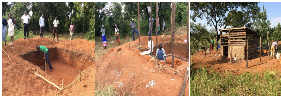
Figure 4: Community involvement in construction of demonstration units
