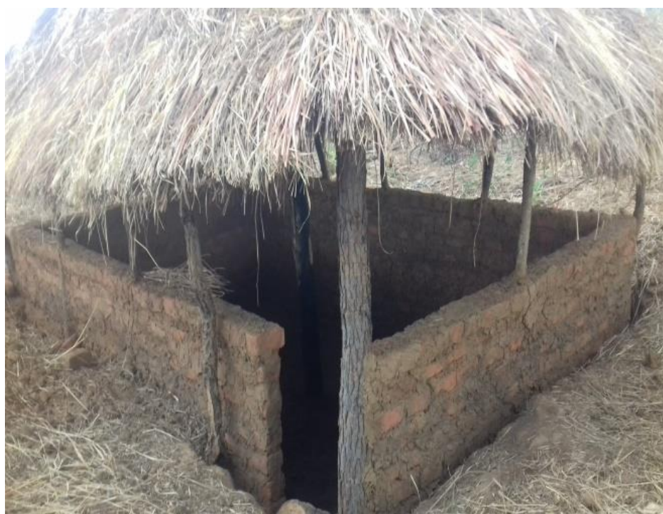
Figure 1. IMO pig house made locally by one of the new pig farmers
