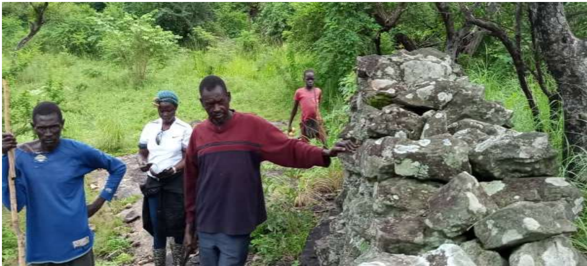
Figure 9: The 0.8m thickness of Gogo stone walls
