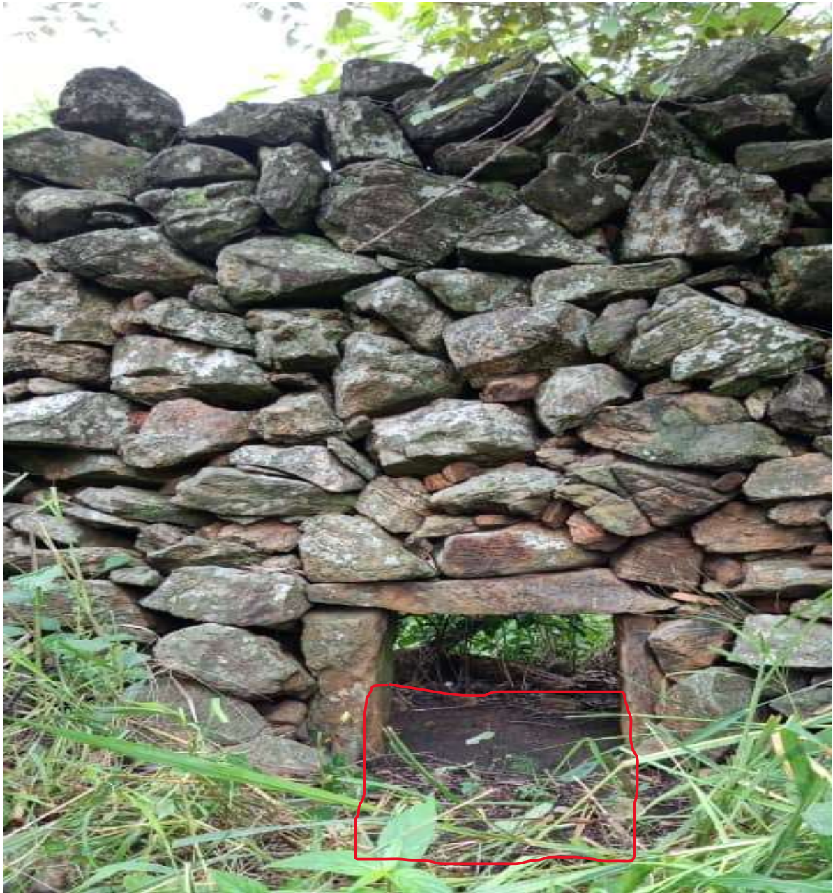
Figure 8: The structure of the opiding at Gogo stone walls
