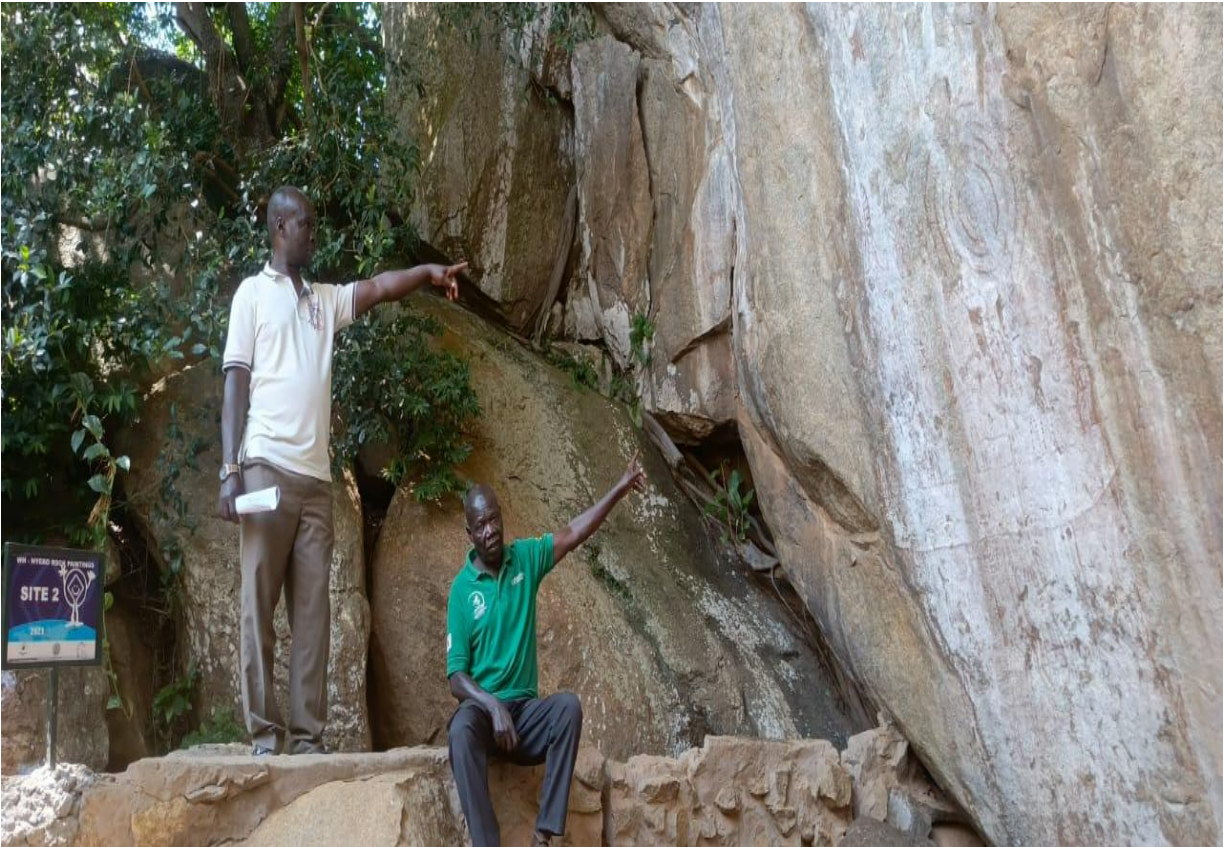
Figure 3: The Researcher with the Tour Guide at an area physically damaged at the site due to weathering
